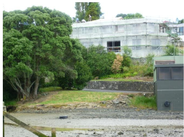
Photograph 8-2 Site with pump station to the right of image
