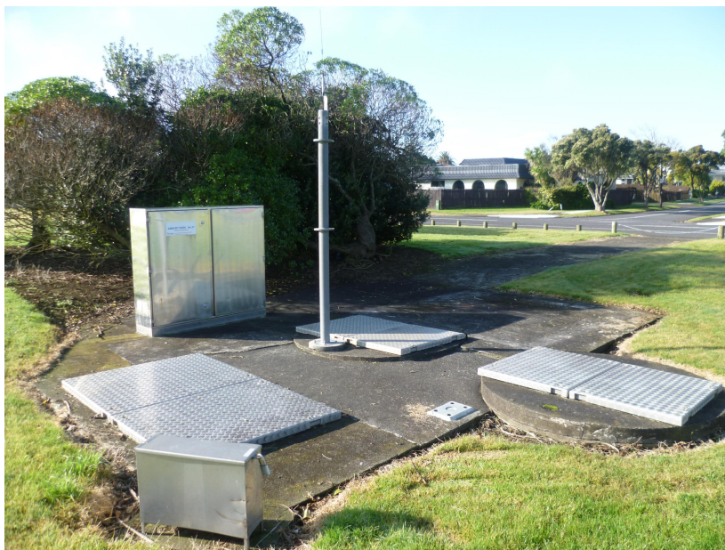
Photograph 9B-1 Existing pump station structures
