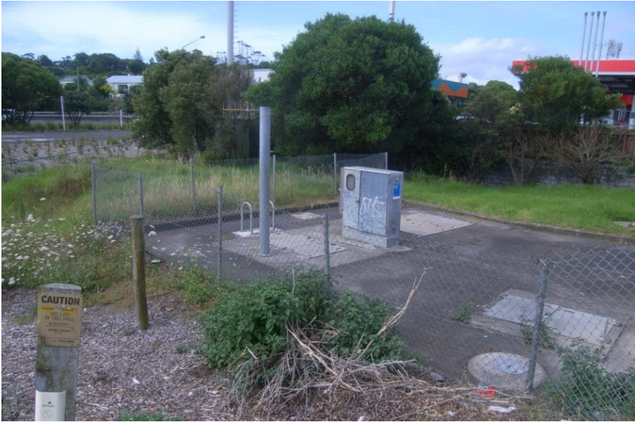
Photograph 1B-1 Construction area
