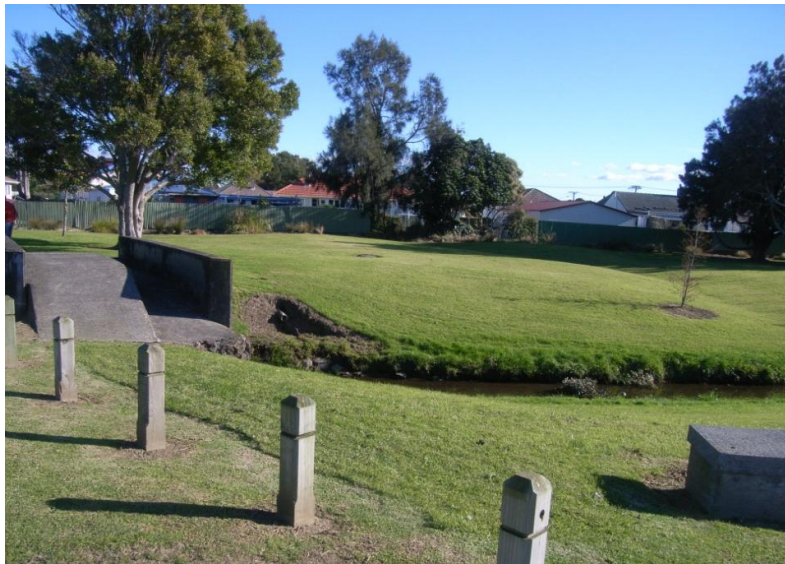
Photograph 5-1 Walmsley Park construction site, facing west
