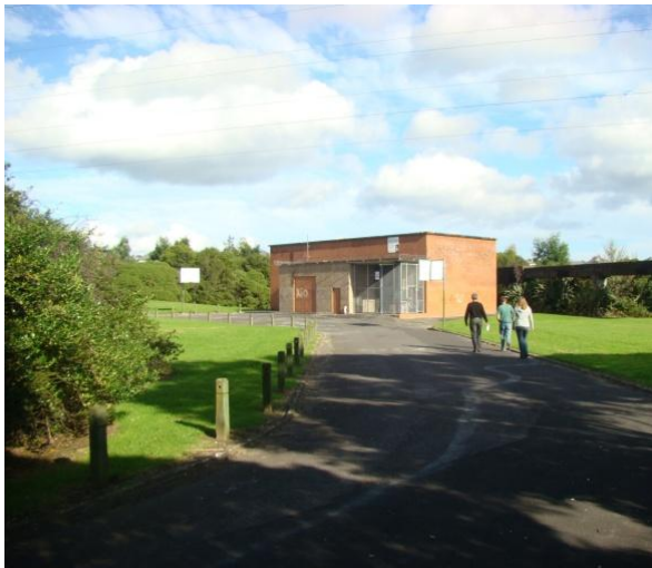
Photograph 15-1 Construction area, showing existing pump station building and above ground sewer
