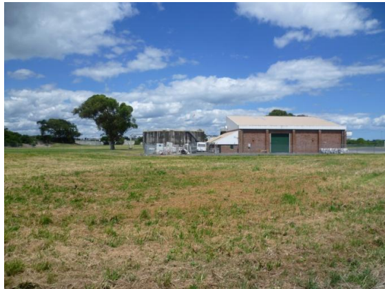
Photograph 10-1 Existing buildings in site construction area
