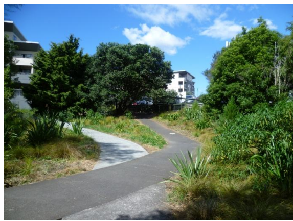
Photograph 3-2 Construction area looking north towards Morning Star apartments
