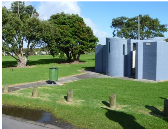
Photograph 9A-1 Existing toilet block within proposed construction area
