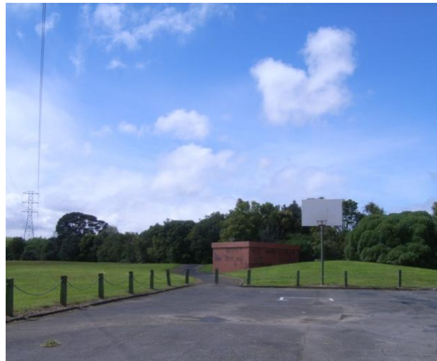
Photograph 15-2 Existing valve chamber
